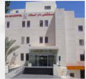
Dar Al Salam Hospital Project - EGYPT
