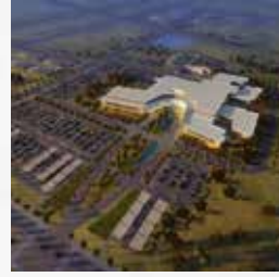
Ministry of Health Project - QATAR
