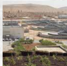
Alsamra Biosolid Monofill Project - JORDAN
