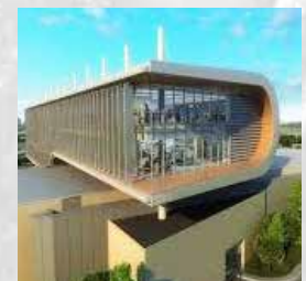
Moro 1.2 Dubai Project - UNITED ARAB EMIRATES
